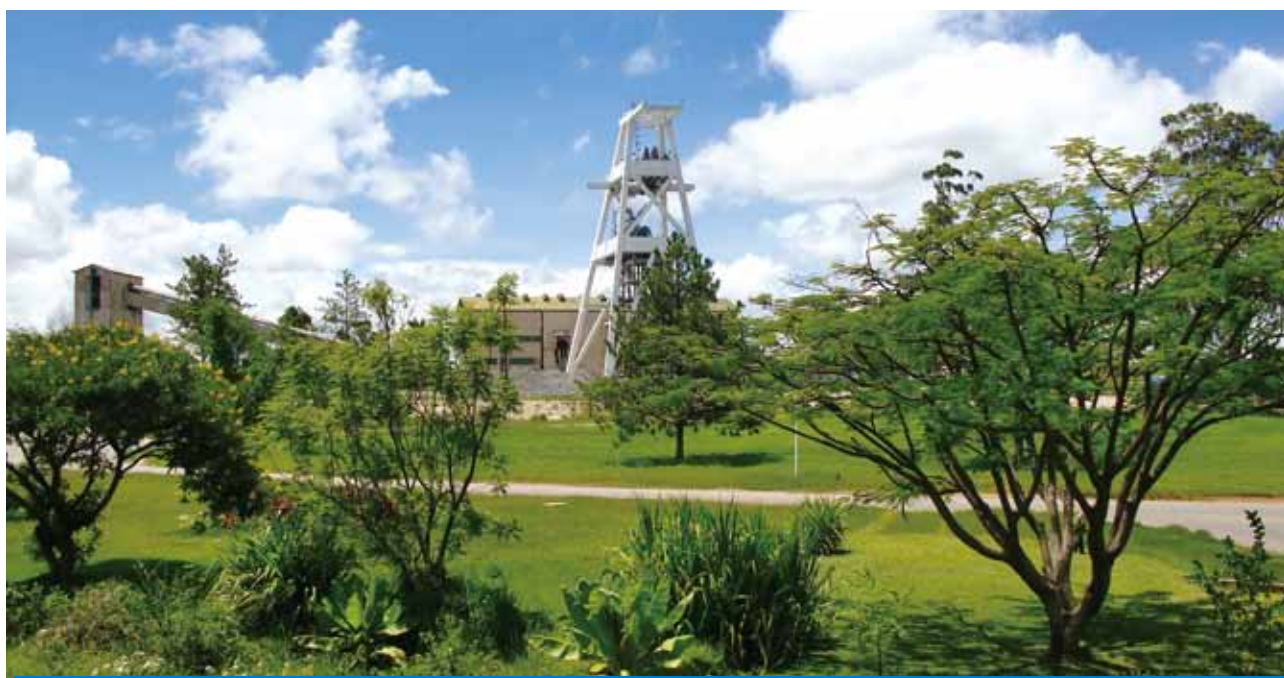
Chambishi銅礦主井架
