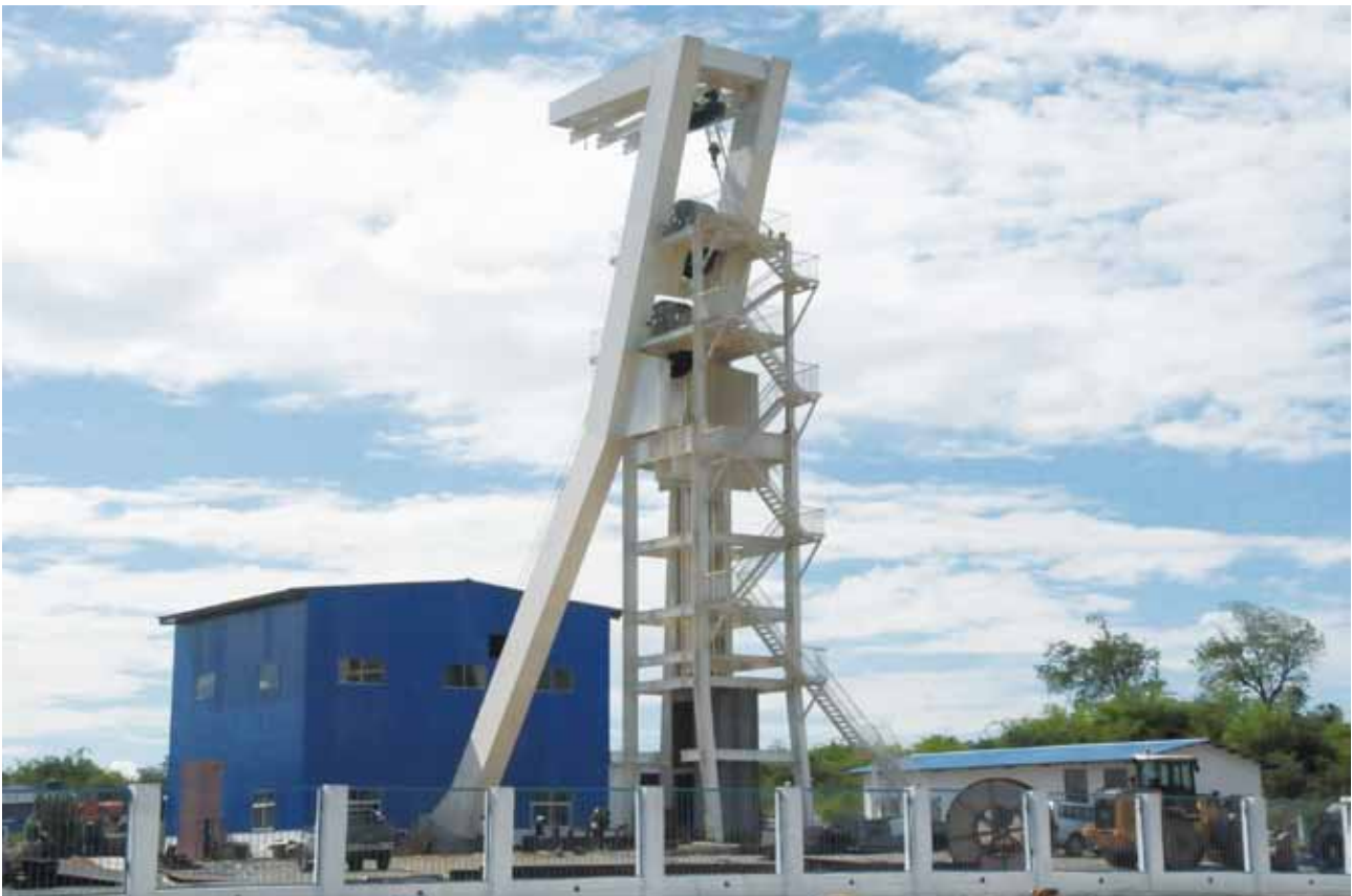
Central auxiliary shaft of Chambishi West Mine
