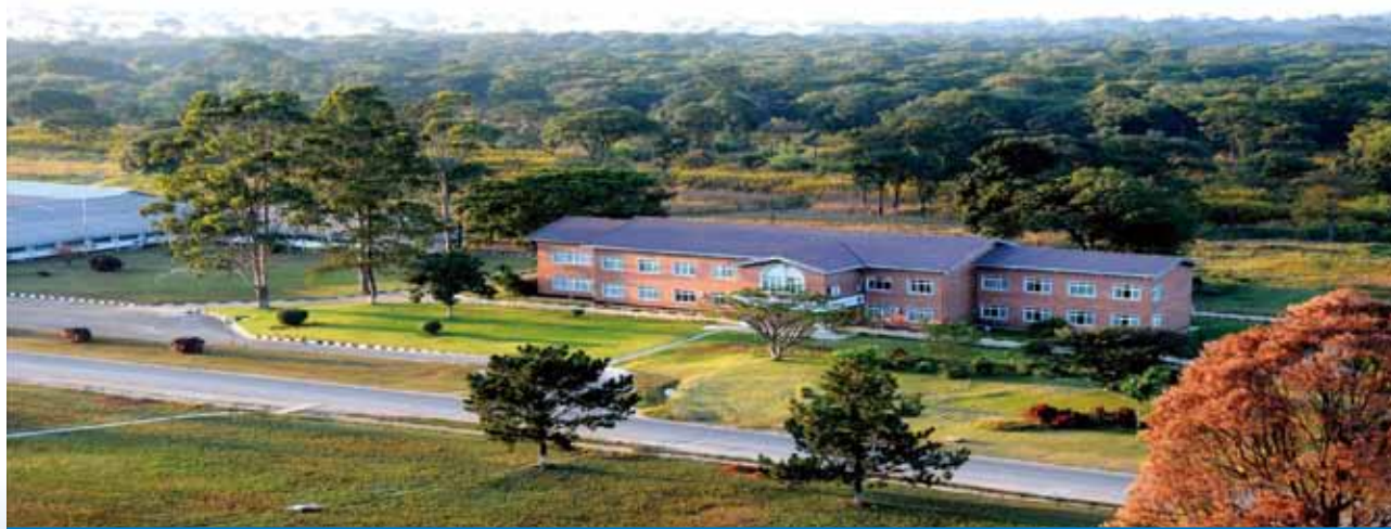
Central office building of NFCA in the green bush
