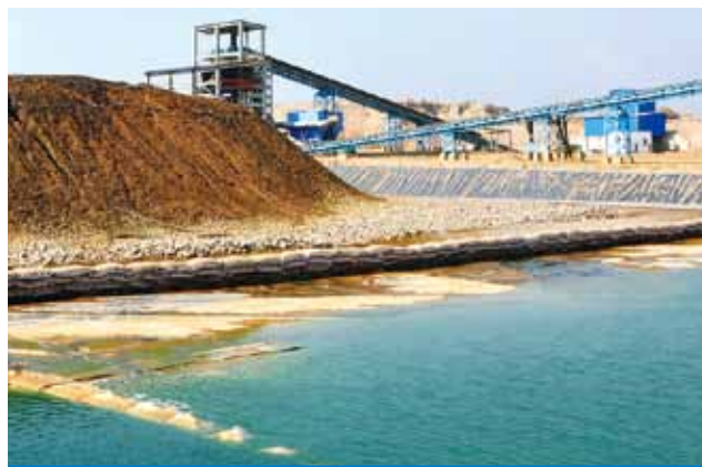
Leach solution from spray leaching of Muliashi Project
