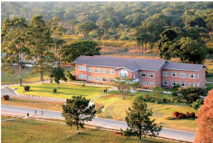
NICA office area
