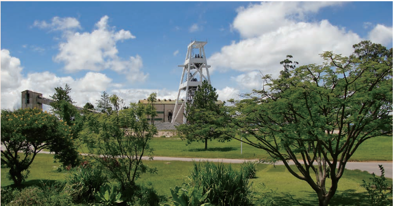
Central auxiliary shaft of Chambishi West Mine
