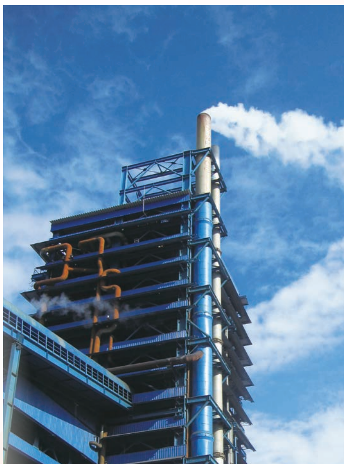
ISA furnace of copper smelting company
