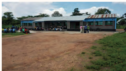
Newly repaired school buildings
