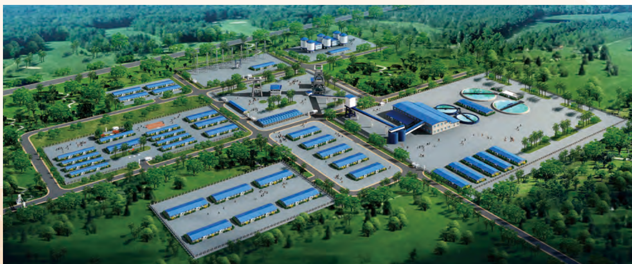
A bird view of the mining and processing project of Chambishi Southeast Mine
