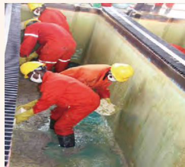
Electrowinning cell overhaul and cleaning
