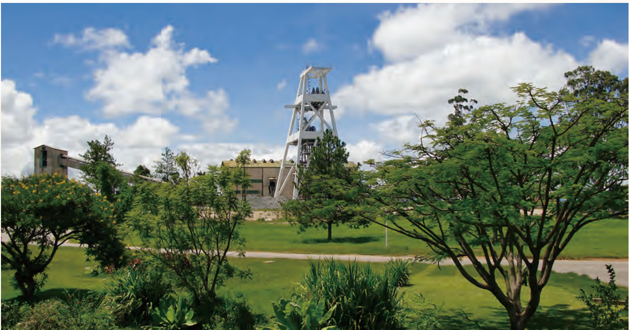
Central auxiliary shaft of Chambishi West Mine
