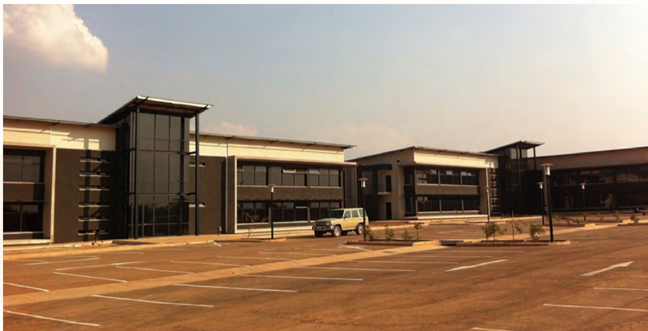
CNMC Huachin Mabende Office area in Lubumbashi in DRC
