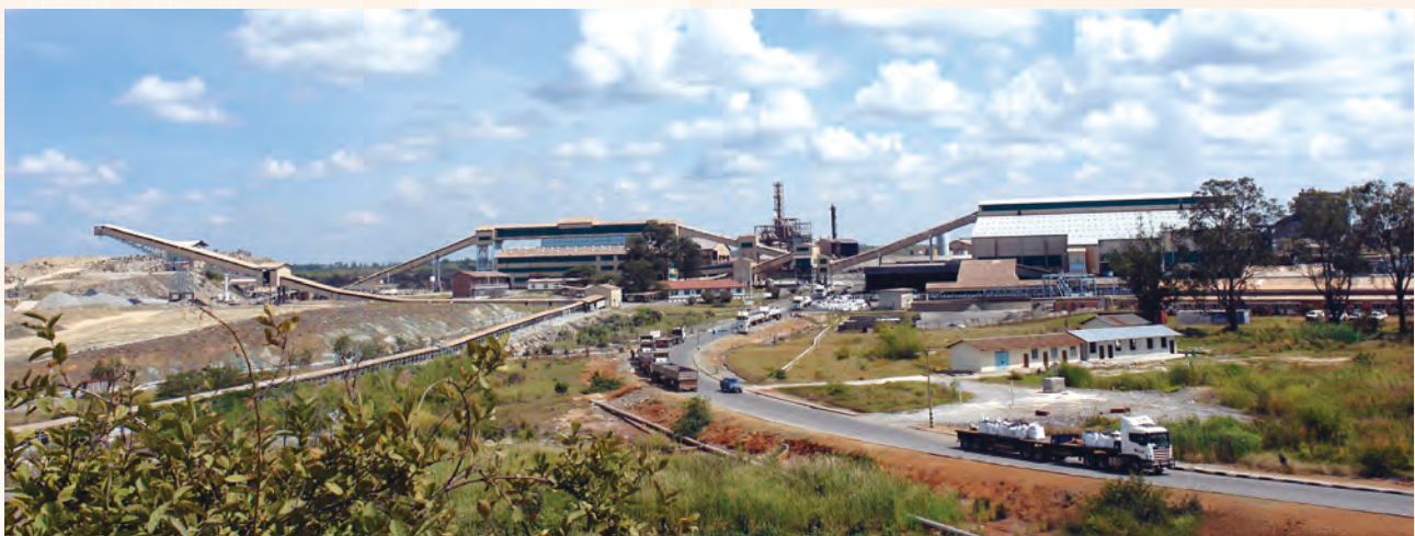
Panorama of Chambishi Copper Mine processing plant
