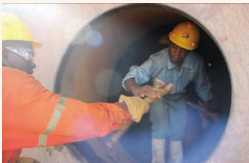
Acid leach tank overhaul and cleaning
