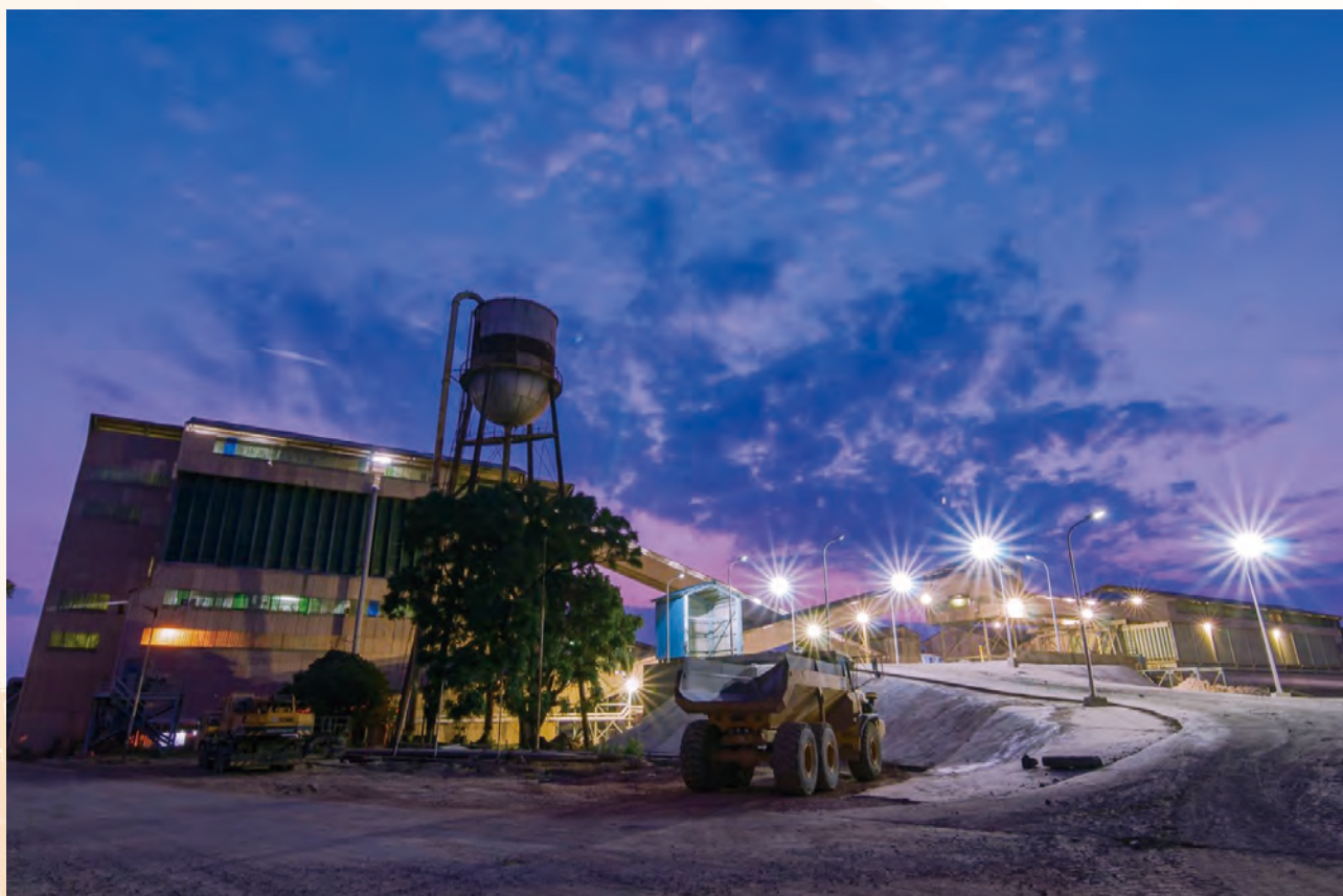
CNMC Luanshya Processing Plant at Dusk
