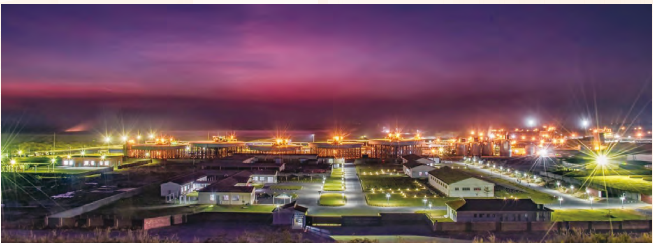
CNMC Luanshya Muliashi Leach Plant at Night
