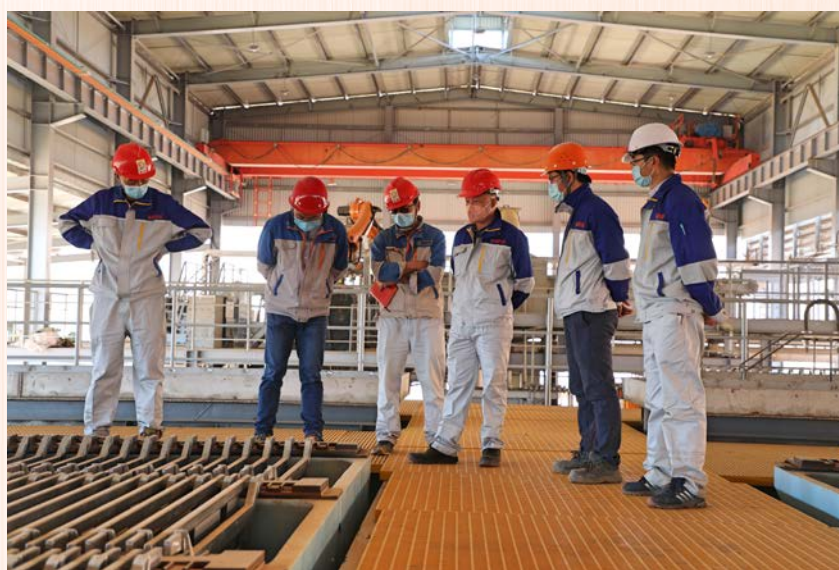
Kambove Mining extraction electrowinning workshop
