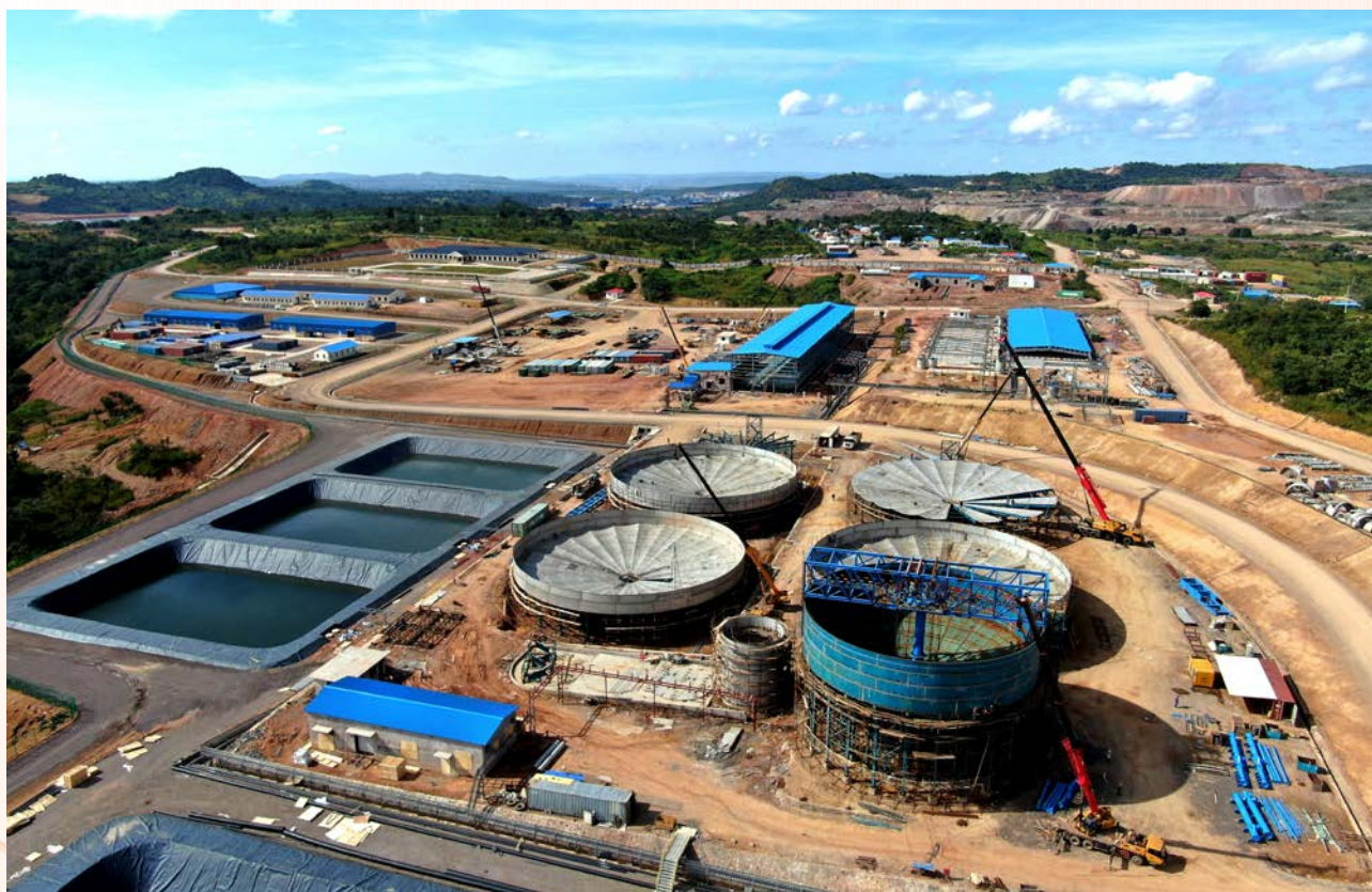
Kambove Mining leach plant construction site
