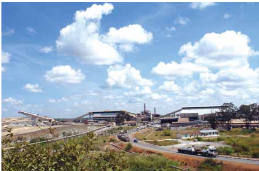
Chambishi銅礦選礦廠全景
