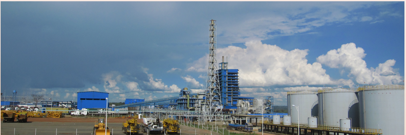
CCS smelting system
