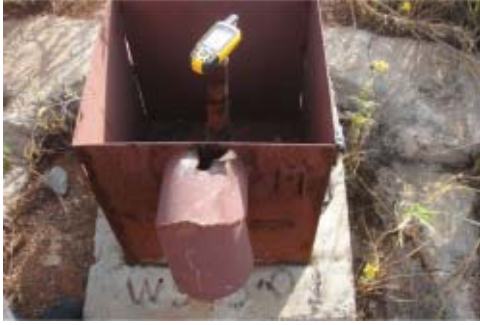
Figure 6-12: Location of Borehole WS001 — Chambishi West Mine
