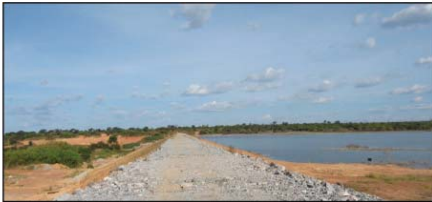
Figure 12-2: NFCA Water Reservoir
