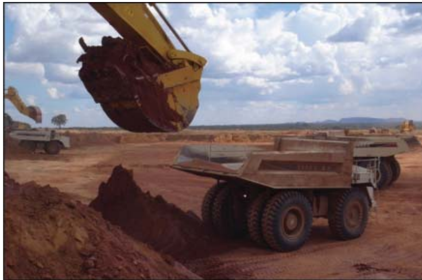
Figure 7-11: An Overview of Waste Loading at Muliashi Northwest Open-pit
