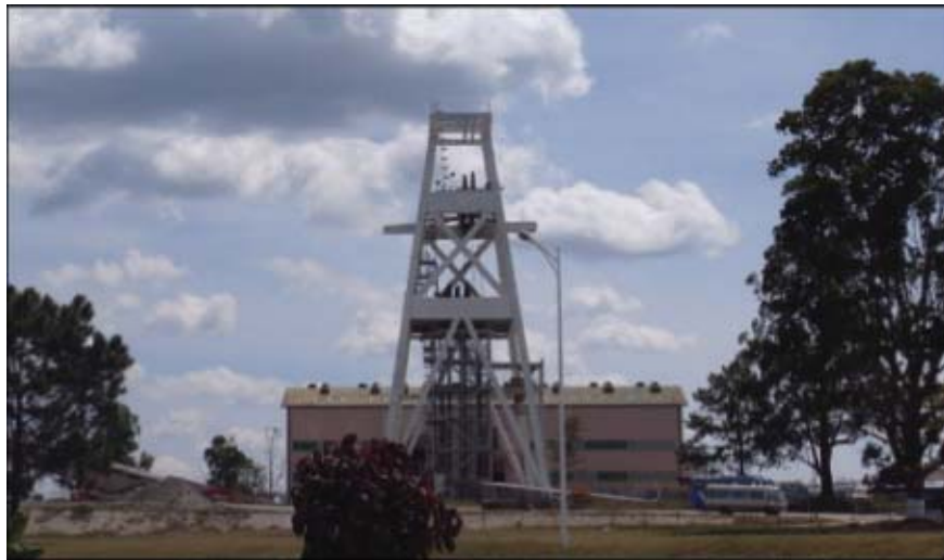
Figure 7-2: An Overview of Shaft 3# at Chambishi Main Mine
