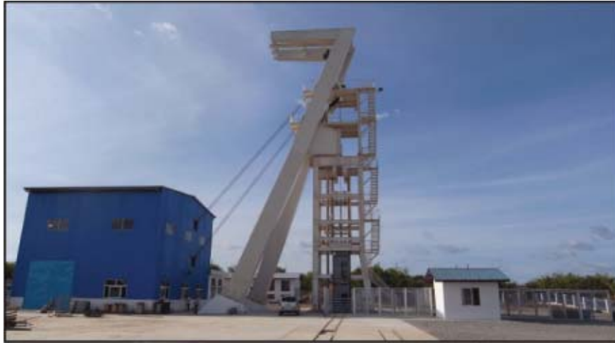
Figure 7-4: Headframe of Central Auxiliary Shaft at Chambishi West Mine
