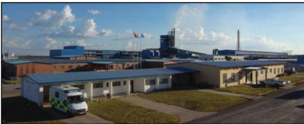
Figure 8-11: An Overview of Chambishi Copper Smelter
