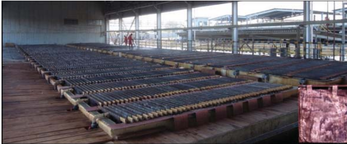
Figure 8-8: Copper Electrolysis Plant
