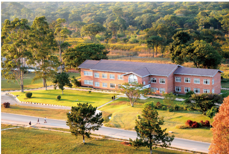
NICA office area
