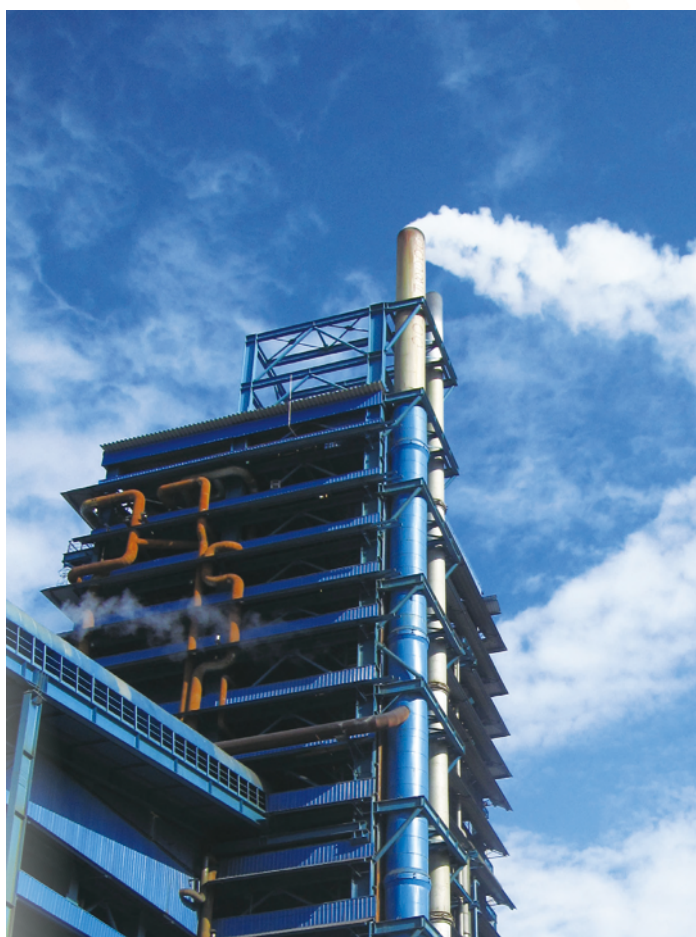
ISA furnace of copper smelting company
