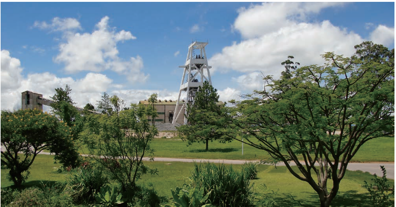
Central auxiliary shaft of Chambishi West Mine
