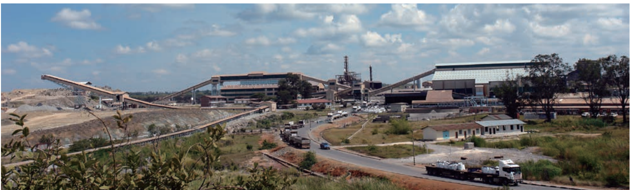
Panorama of the ore processing plant of Chambishi Copper Mine
